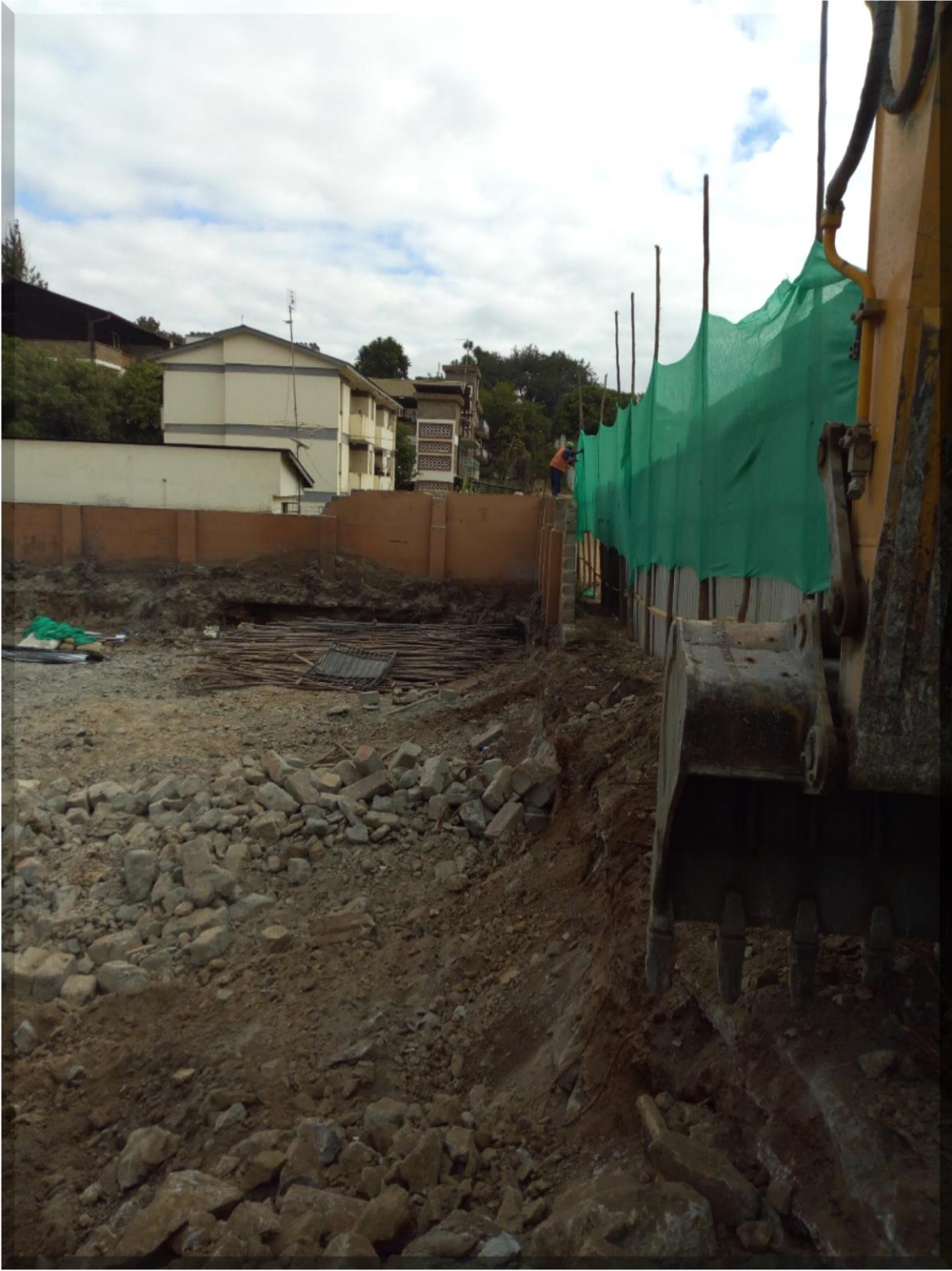
Fig. 05. Excavations works progressing on as below
