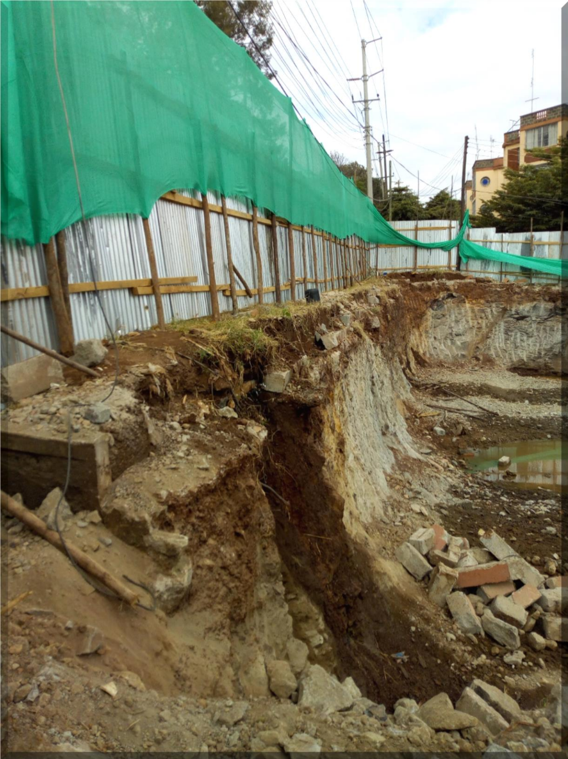
Fig. O6. Excavations works progressing on as below
