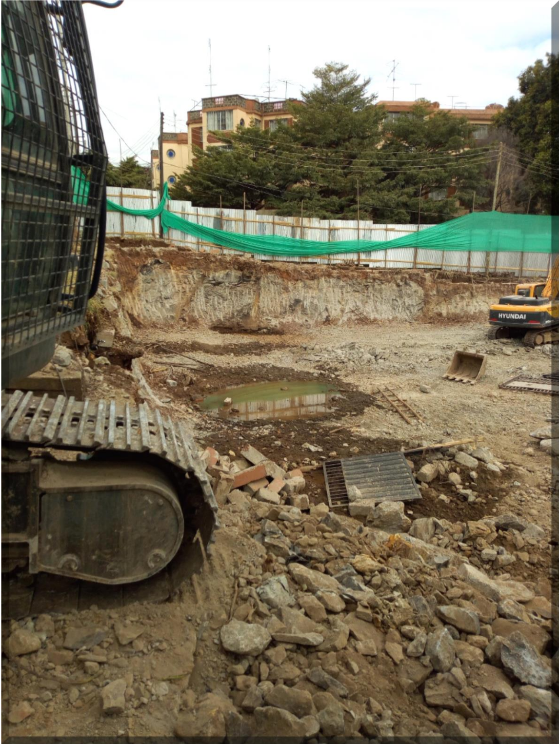
Fig. 02. Excavations works progressing on as below
