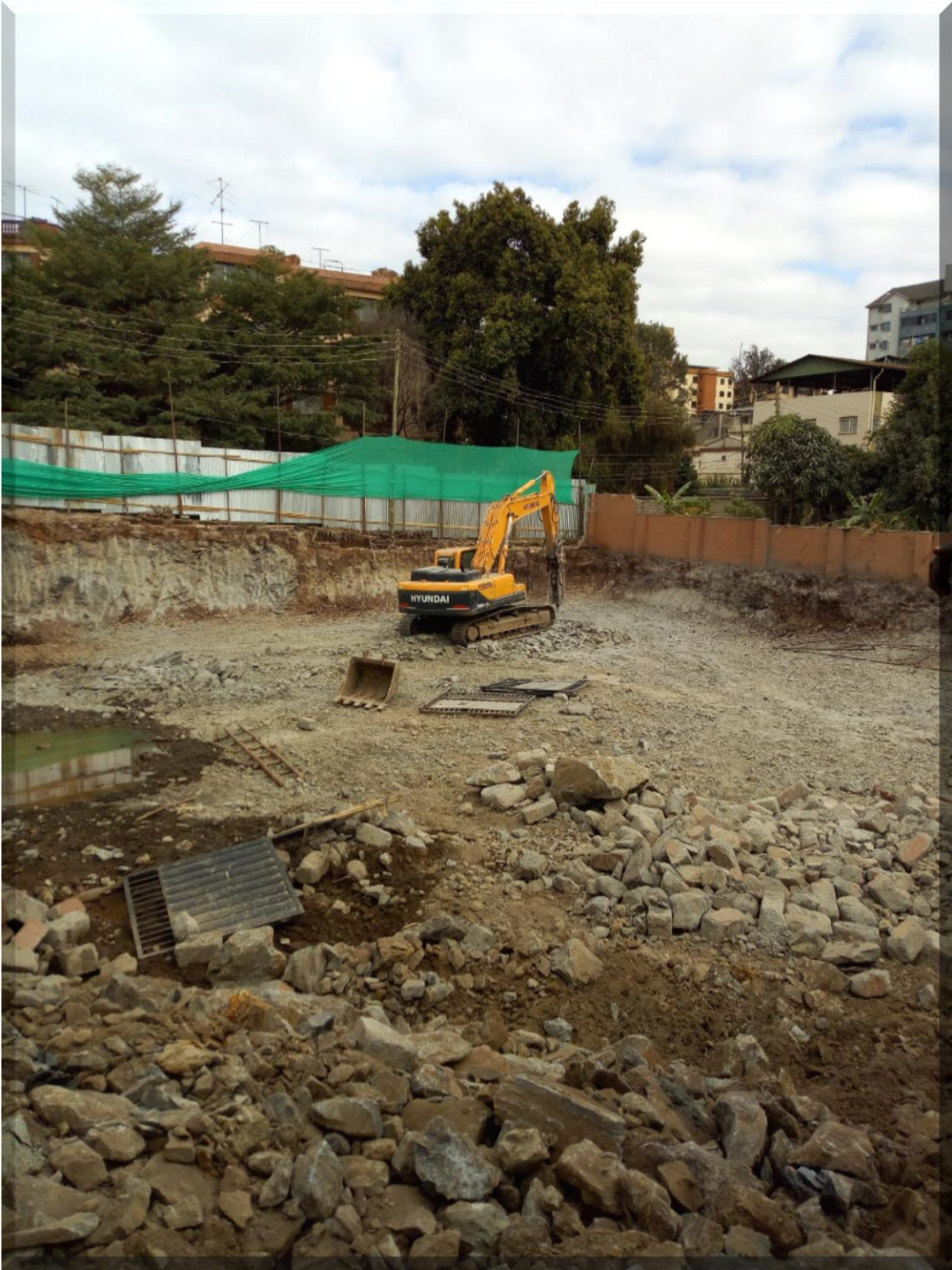
Fig. 03. Excavations works going on as below
